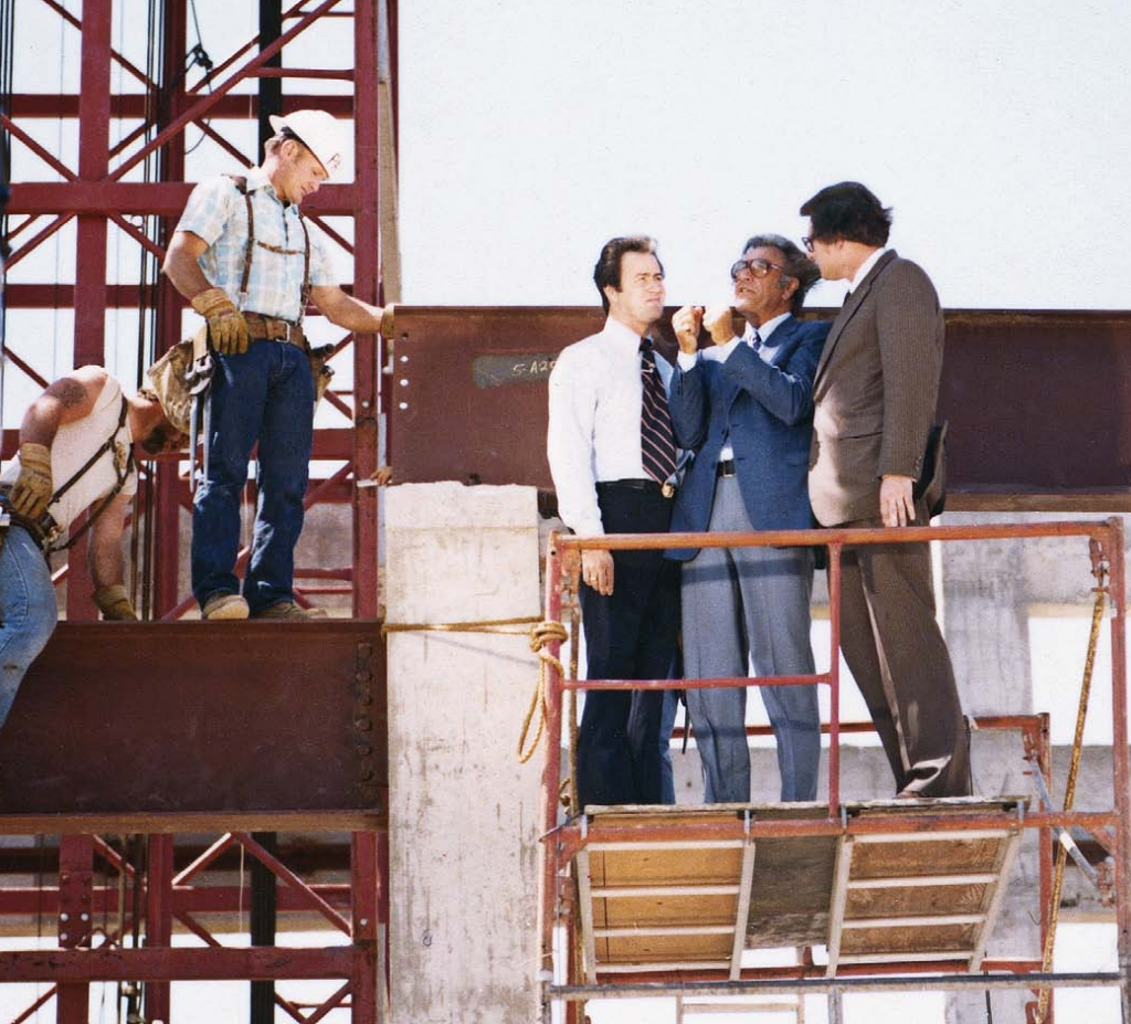
Oral and Richard Roberts along with Dr. Jim Winslow at the City of Faith construction site.
